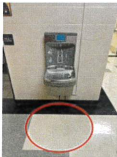
HS hallway. Recommend installing floor mats in front of drinking fountains to prevent slip and falls
